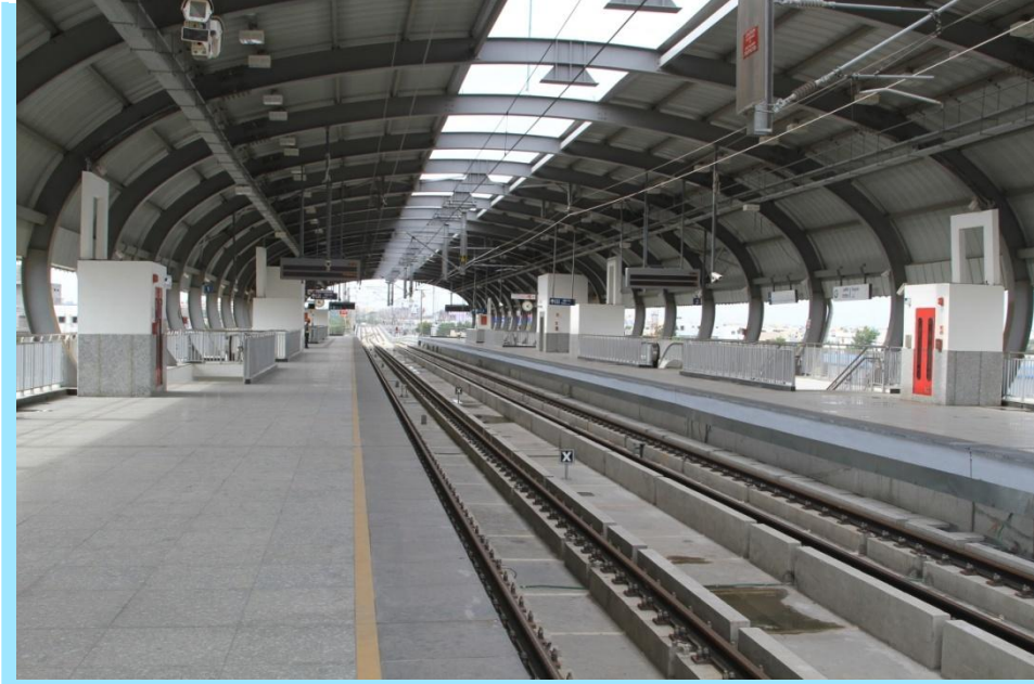
Platform level of Metro Station
