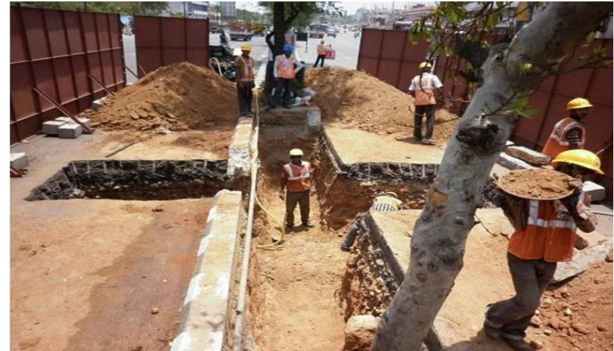
Soil Load Test being done before constructing Metro Rail Pier
