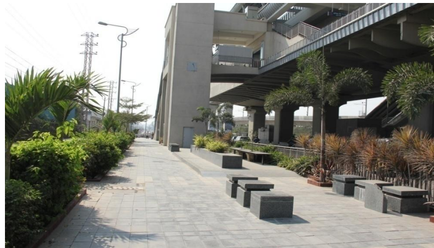
Streetscaping, Parking & Pedestrian facilities, etc., at Nagole Metro station
