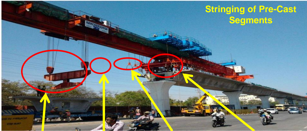
Traveller For Lifting and Shifting Segments
