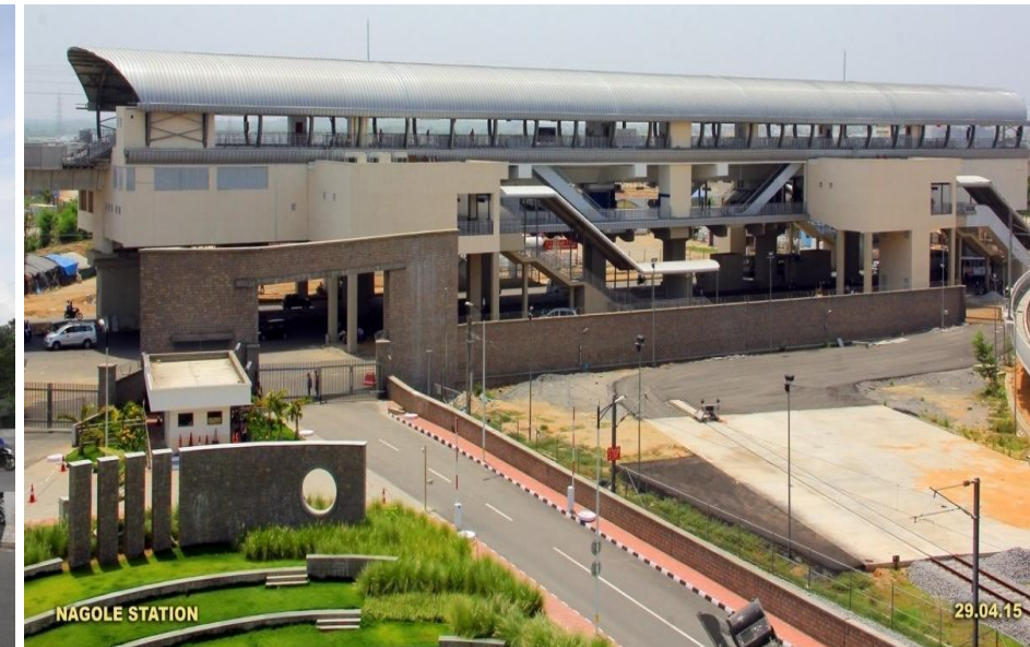
Metro Rail station-Lateral View
