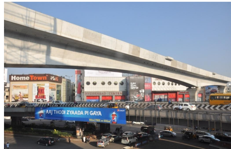
Metro Viaduct crossing flyover
