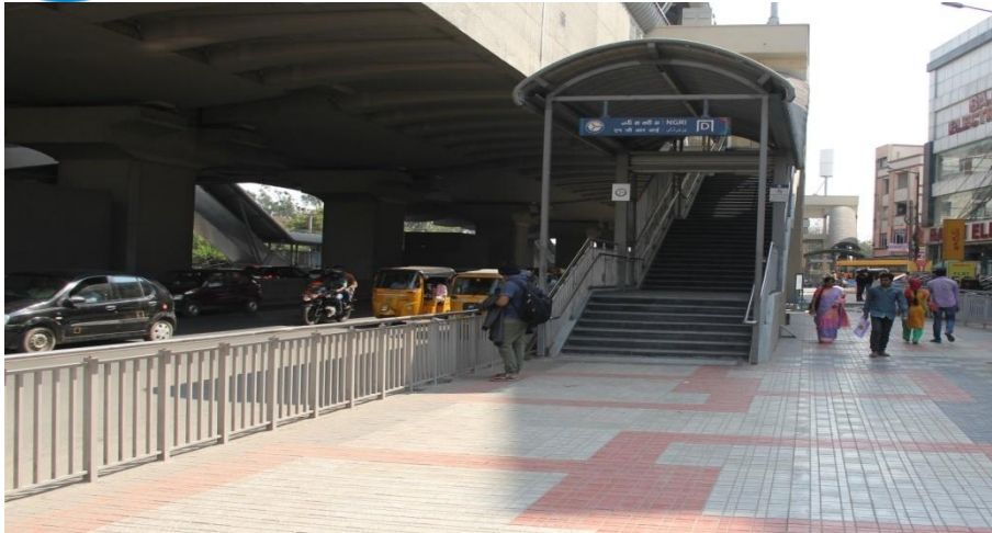
Streetscaping, Parking & Pedestrian facilities, etc., at NGRI Metro station
