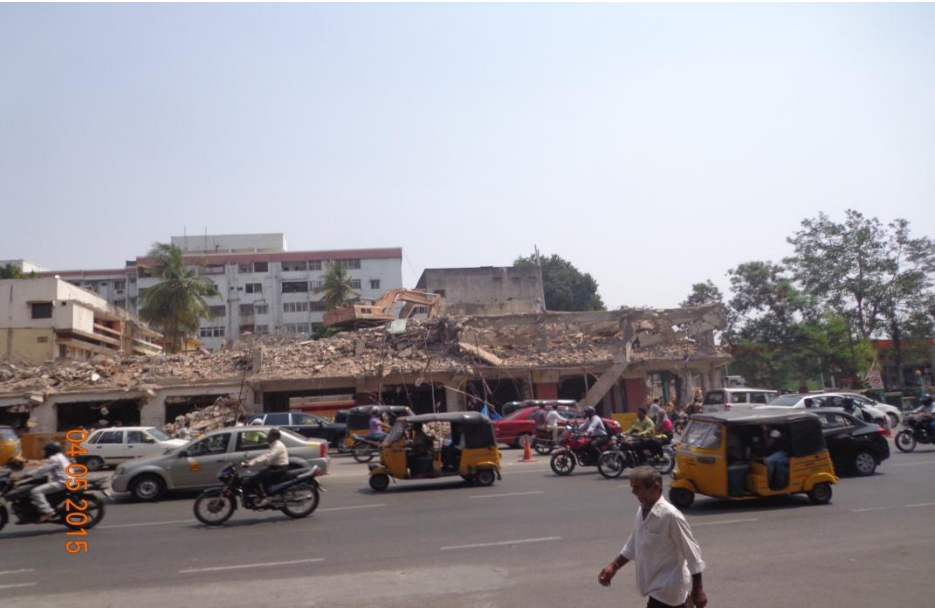
Demolition of Jabbar building
