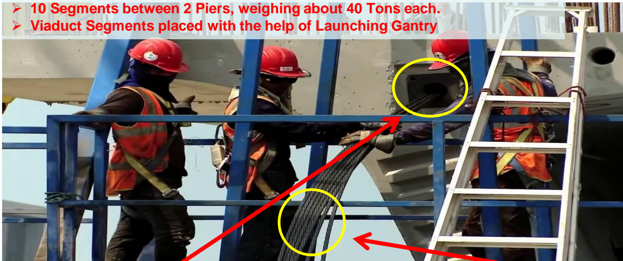
Duct in Pre-Cast Segment
