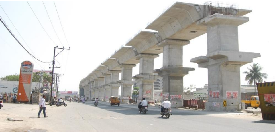
Metro Station Construction-Pier & Segment Stage
