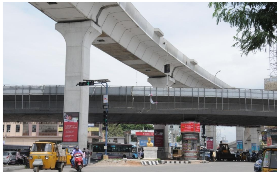
Metro viaduct crossing at Malakpet flyover
