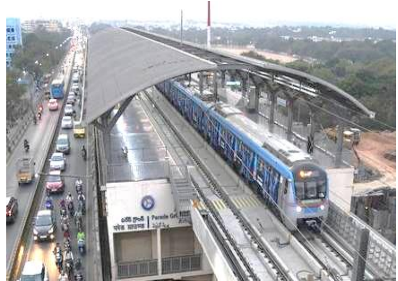
Hyderabad Metro Rail - Typical station
