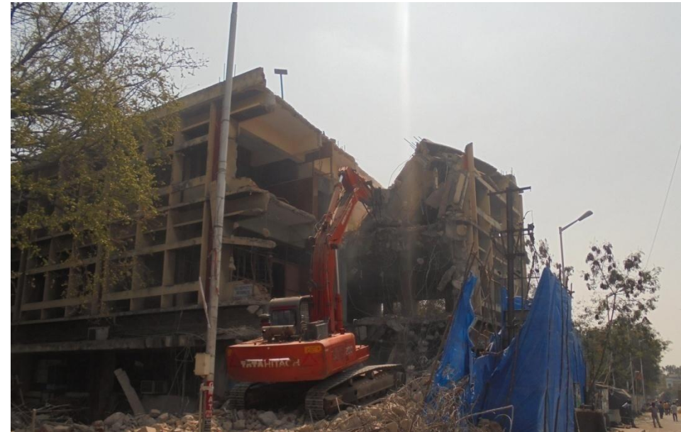
Demolition of BHEL building
