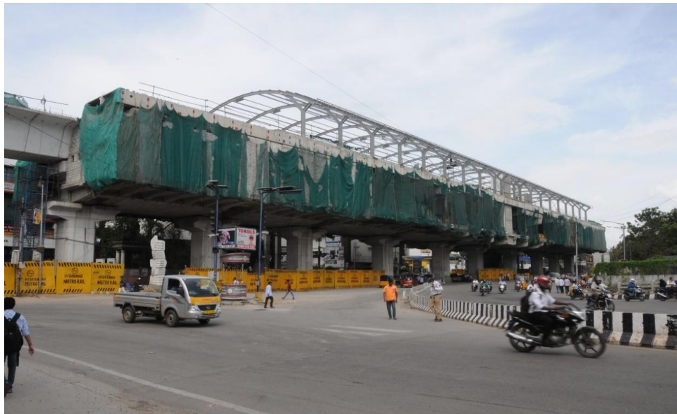
Metro Station Construction-Roofing Stage
