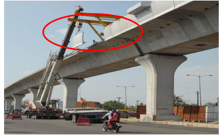
Erecting Parapet Wall on the Viaduct
