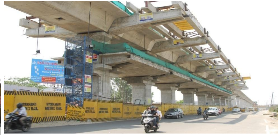
Metro Station Construction-Spine & Wings Stage
